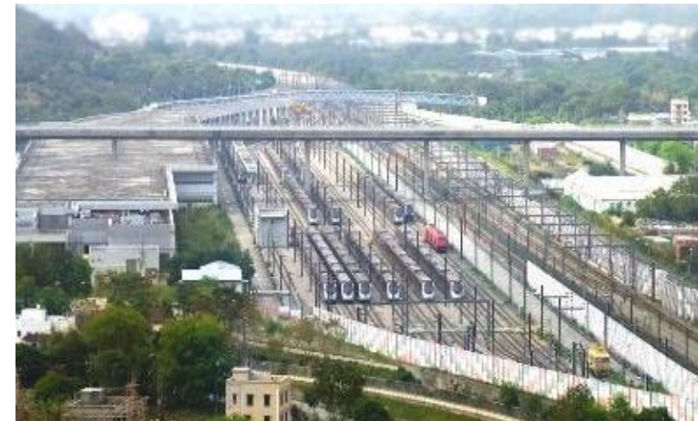
Interface with Operating Railway
